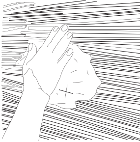
Applying layers of plaster
